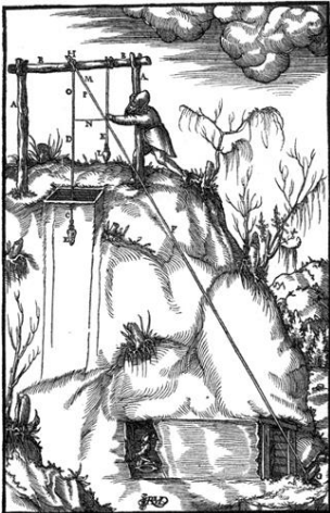
Fig. 8 Connecting survey and orientation measurement according to Agricola [3]
