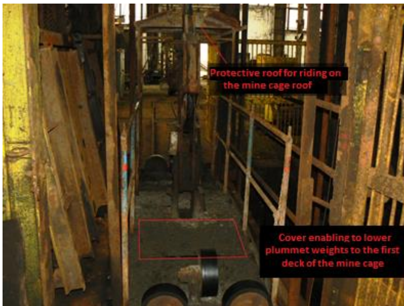
Fig. 29 Mine cage roof
